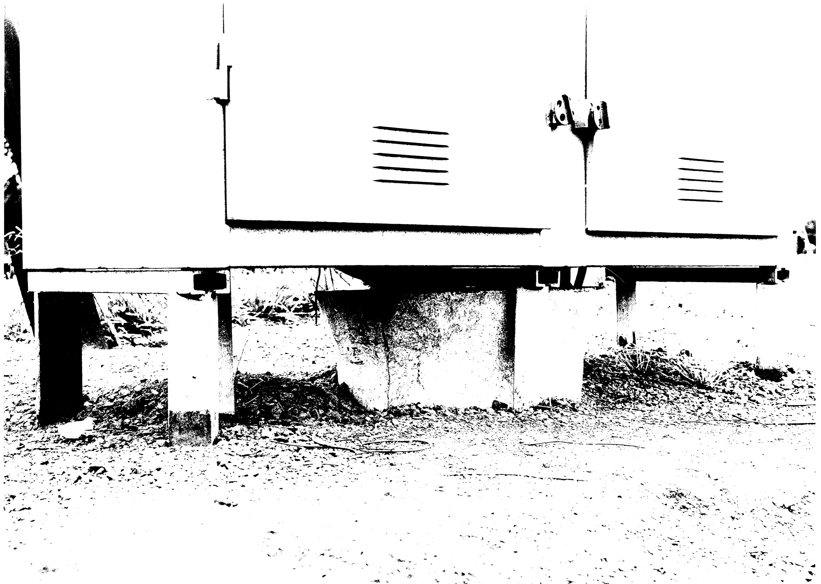
CABLE PIT MOUNTED UNDER RELAY BOX
