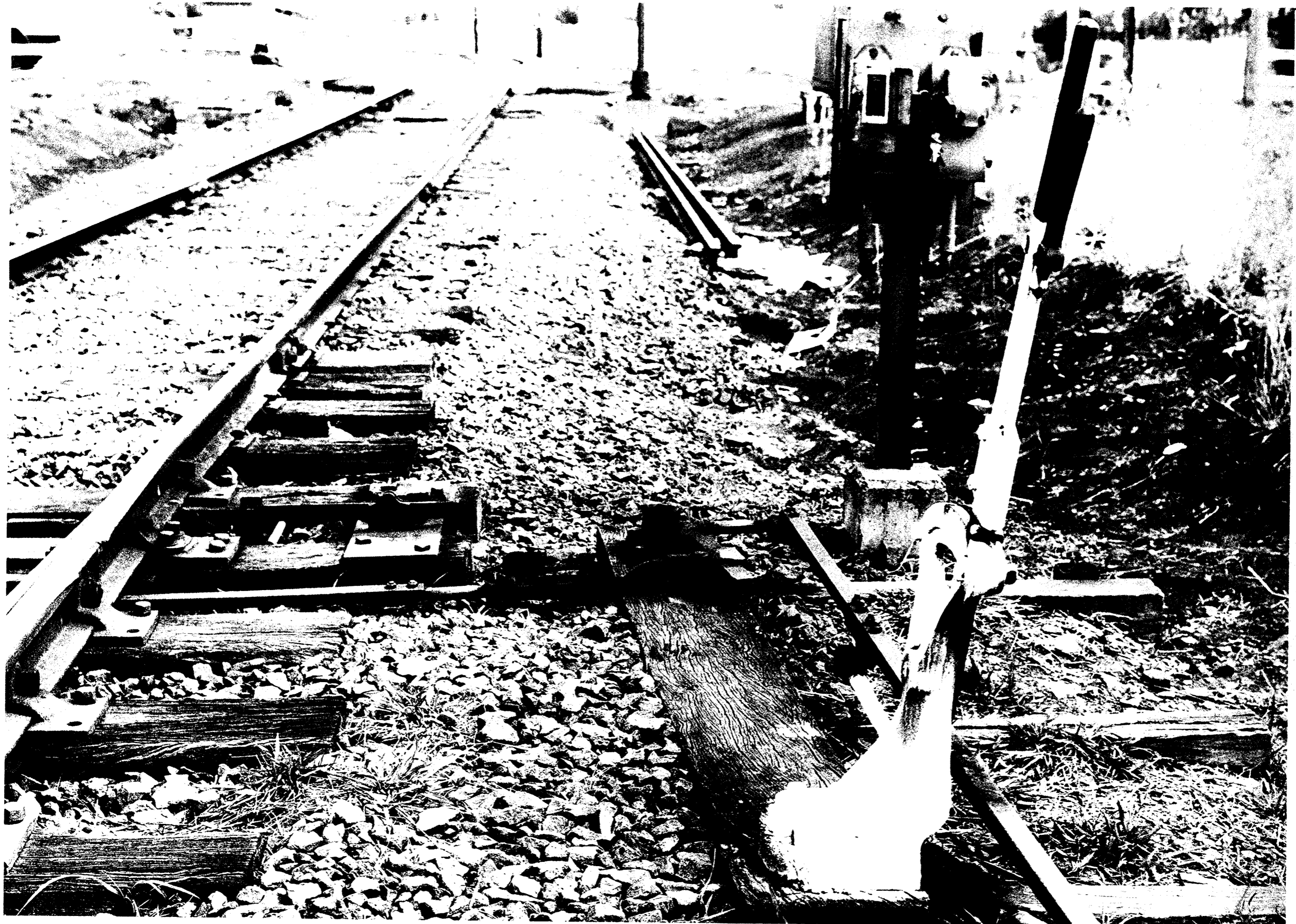
ANNETT LOCK POINT LAYOUT AND LEVEL CROSSING PUSH BUTTON CONTROL.
