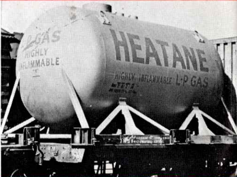
Liquid petroleum gas container.
