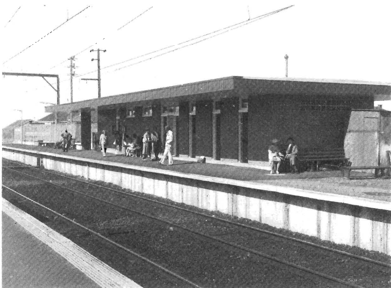
Moorabbin station, a new building was necessary to fit in with the third track project between Caulfield and Mordialloc.
