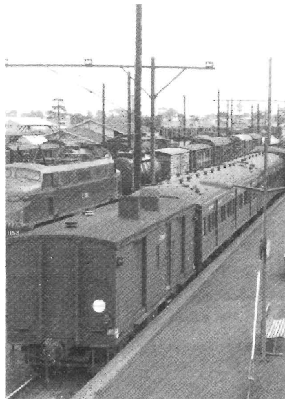
Dandenong station got a facelift with a new platform that protects passengers.
