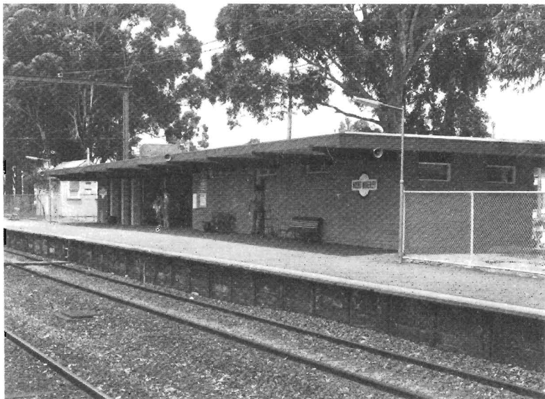
Mount Waverley station, rebuilt as part of the upgrading of the Glen Waverley line. The subway has been decorated with a mural, painted by college students.
