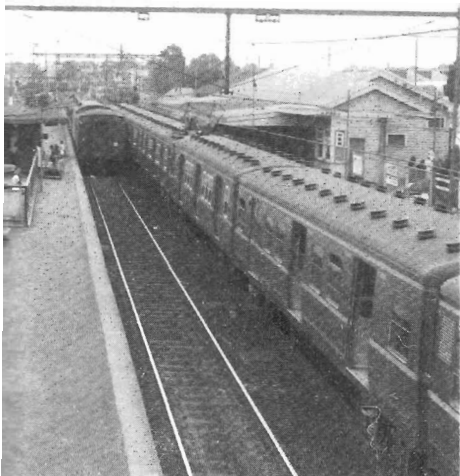
...coat of paint. And a brick shelter (on the left) ...ing on platforms 1 and 2.
