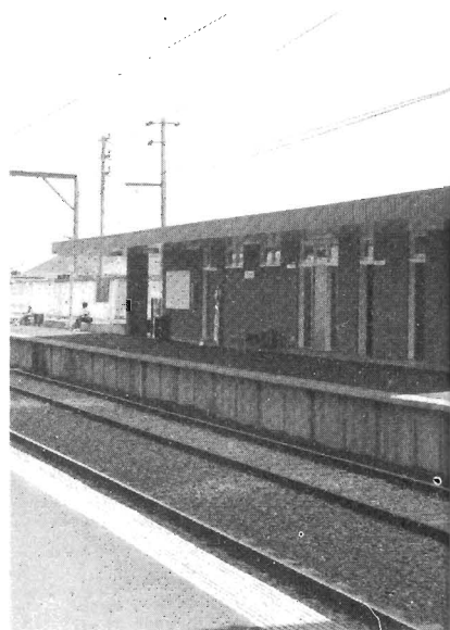
Ormond station on the Frankston line. The new platform is a model as part of the third track project.
