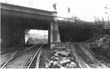
Progress on the Footscray quadruplication is now centred on approaches to the Hopkins Street bridge. On the Williamstown line side (above), the bridge approach has been prepared, while on the St. Albans line side, workmen are blasting their way through the bluestone. Space for one of the tracks from South Kensington has also been finished and the embankment sprayed with concrete to stabilise it. Work will start soon on cutting the way for the track to come through on the south side.
