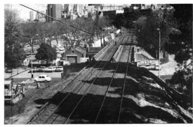
Between Jolimont station and the city, work is progressing on building a retaining wall and widening the railway formation to take a third track. Recent bridge works over Jolimont road made provision for the third line.
