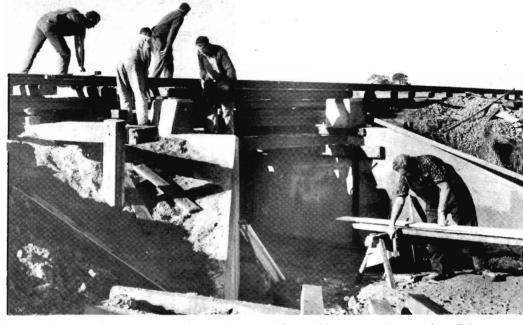
LITTLE BRIDGES are also part of the railway scene. Here, at Myamyn, workmen are busy lining up a small concrete culvert.
