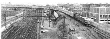
At North Melbourne, the retaining wall alongside the flyover has been completed as has the base of the ramp. Southern Aurora can be seen going over the new opening in the flyover. The approach ramp on the other side of the flyover is also completed.
