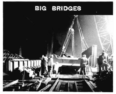
Bridge building was big news during July. In another week-end battle against fog and time, railway workmen positioned a pre-fabricated steel bridge structure at Francis Street, Yarraville. During the early hours of the morning, when the fog lifted a little, this was the scene as workmen guided the bridge into position.
