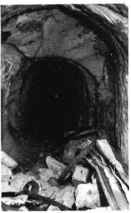
No bracing was needed inside the small diameter tunnels. This one extends for over 300 yards (274 m) according to locals.
