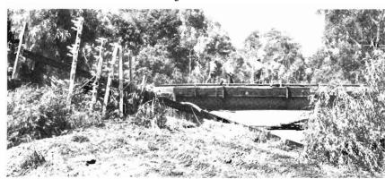
COMMUNICATIONS WERE CUT when four poles were washed out. The poles carried communications and signals power and circuits. Emergency arrangements to keep trains running in the unaffected areas were achieved by using P.M.G. telephone circuits and local S.E.C. power.
