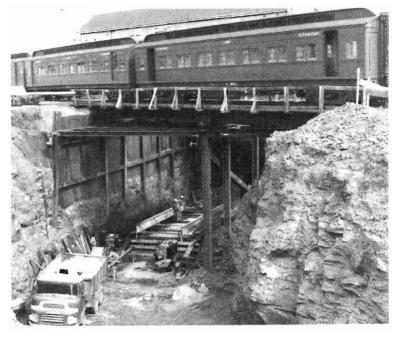
Tunnelling in the Spencer Street area extends from the pilot tunnel under La Trobe Street, under the rail tracks leading to the country platforms, and will soon move into the area near the suburban platforms. At one point, the twin tunnels pass underneath the corner of No. 1 Signal Box, which is temporarily supported while construction continues underneath
