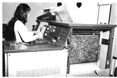
Data Processing Assistant, Michele Healy, uses the 1004 Electronic Data Processer before it was released on delivery of the new G 415 computer. Programmes for the 1004 were the maze of wires inserted on a panel (at right).
