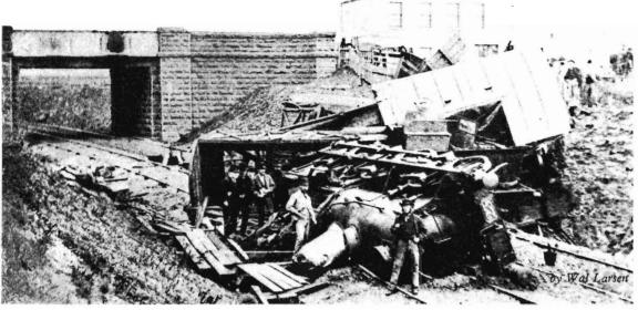
On August 23, 1873—one hundred years ago—a train left the Geelong goods shed behind locomotive 0 23. However its planned journey came to an abrupt halt about 1.6 km (one mile) out when the locomotive's boiler exploded.
