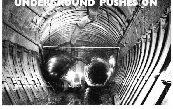
The shape of things to come—Codelfa Constructions Pty. Ltd's. tunnel under Spring Street which, in a few years, will see trains instead of construction vehicles in its 6.7 m (22 ft.) diameter tunnels.
