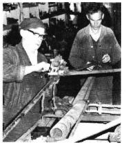
Don Mason (left) and Bill O'Loughlin go about their task of renovating a pantograph from a metropolitan train. An average of two pantographs are completely restored each
