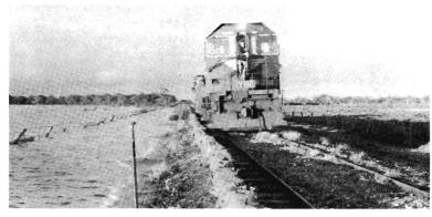
One of the key areas protected was Foster's Swamp along the Kerang-Koondrook line. This photograph of the sandbag train shows the levee along the railway ready to stem the water from crossing it into Foster's Swamp. The permanent levee is just on the other side of the submerged fence. Water reached to within 12 mm (half an inch) of the top of the levee along the railway.
