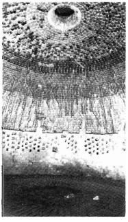
Inside a bottle kiln. Designed to distribute heat and glazing evenly, up to 1,300 products remain inside the kiln for up to four days, while the temperature is brought to 1,200°C. Salt is then added for glazing.
