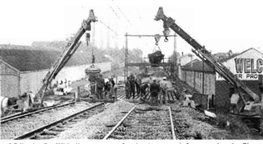
While the St. Kilda line was out of action last month for renewing the City Road bridge, railway workmen also took the opportunity to do a similar – but smaller – renewal at nearby York Street bridge. Here, in 16 hours, new beams and decking replaced the old, concrete was poured and the tracks restored, to give the old bridge a new lease of life.
