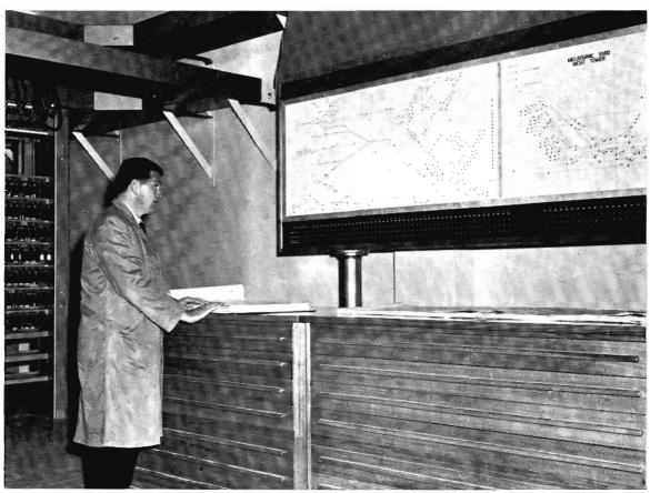
At the signal maintenance diagram in West Tower, Engineer S. White conducts tests from circuit plans. This diagram is a photographic replica of that in the signal box two floors above; it facilitates maintenance work on the system.
