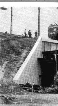
The week-end of August 2 and 3 saw completion of a further stage of the reconstruction of the Swanston Street bridge over the railway lines near Flinders Street station. While the bridge was closed to traffic, old girders, varying from 10 ft. to 44 ft. span, were replaced with new ones. The picture shows a section of old girder and roadway being lifted out.
