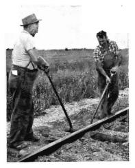
Ganger A. E. Rosenow (left) and Repairer A. J. Davis are packing the track near Rochester.
