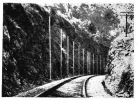
Falling rocks: This fencing along a railway track in U.S.A. emits a signal when struck by falling rocks or earth slides; this also sets the stop signal, and alerts the train controller to the presence of a dangerous situation. ( $Railway\ Age$ )
