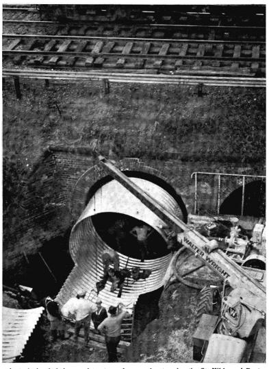
A steel pipe is being used to strengthen a culvert under the St. Kilda and Port Melbourne lines.
