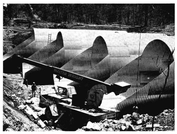
Steel pipes are in position for one of the bridges on the Hurstbridge line.
