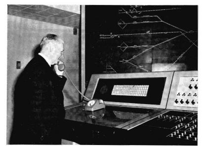
At the opening of West Tower, Block and Signal Inspector V. Bonighton is using the 'phone at the signal box control panel. At the back is a section of the diagram showing what signals are cleared and the location of trains.
