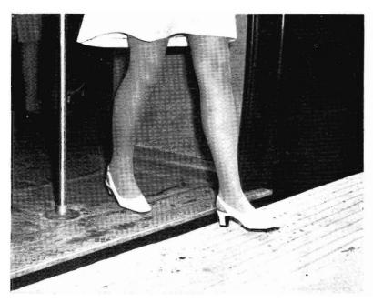
NEW PLATFORM HEIGHT: A passenger alights at the new Canterbury station. This is the first platform to be built with a height of 3 ft. 9 in. above rail level. Where possible, this standard will be progressively adopted when new platforms are provided, when renewals are being undertaken, or when extensive repairs to existing platforms are required.
