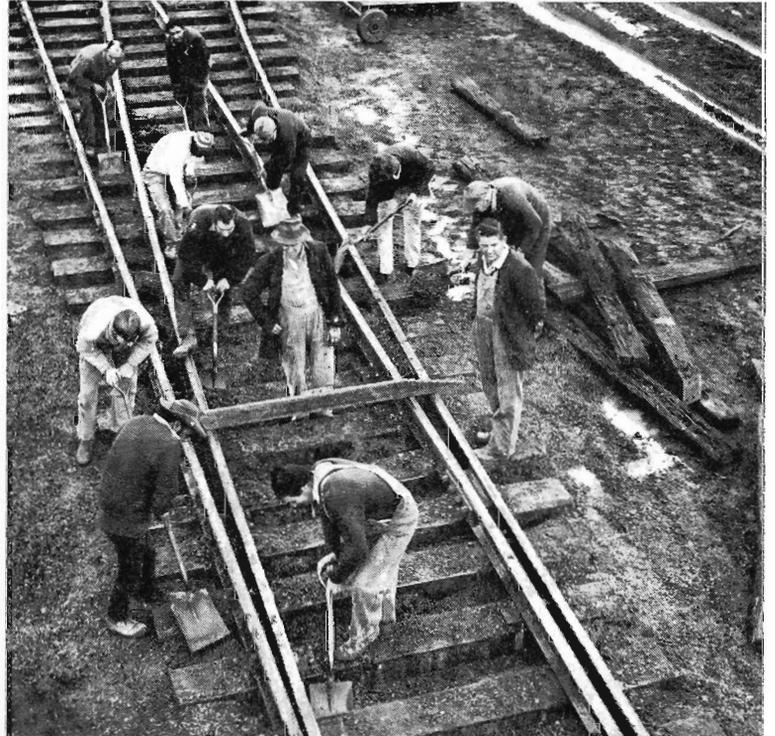
At Portland North, a points and crossings gang, under Special Ganger L. Thompson, is engaged on track alterations for the new terminus.
