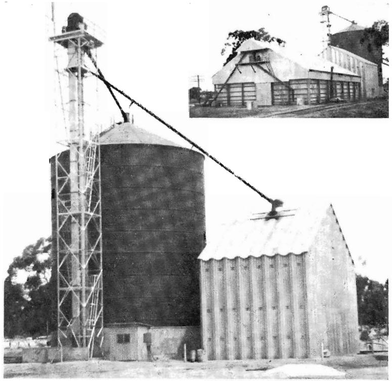
Wheat is received at the steel elevator (left), and passes to the *Behlen* shed used as an annex bin. Inset shows the oats storage bin adjacent to wheat storages.
