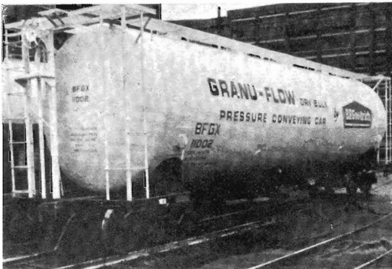
Among special wagons developed in U.S.A. to facilitate bulk handling is this Granu-Flow wagon that has inflatable, rubber-coated diaphragms inside. When inflated, the diaphragms break up compacted loads and channel the contents towards discharge outlets for fast unloading.
