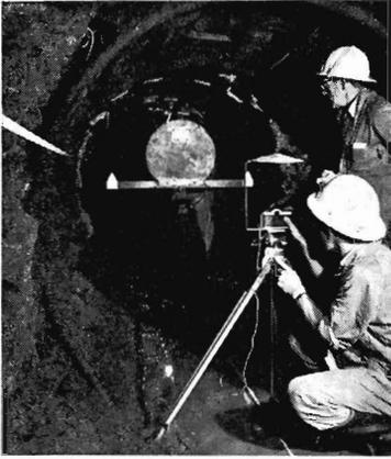
Lining up the camera for a picture. Strips at the sides and bottom are steel measuring tapes. Points on each side of the disc are required for accurate positioning of the subsequent print with the grid.
