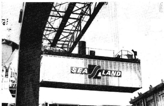
35-ft. Sea Land Containers being loaded onto ship at Elizabeth, New Jersey. Note special frame that is attached to top of container for lifting.
