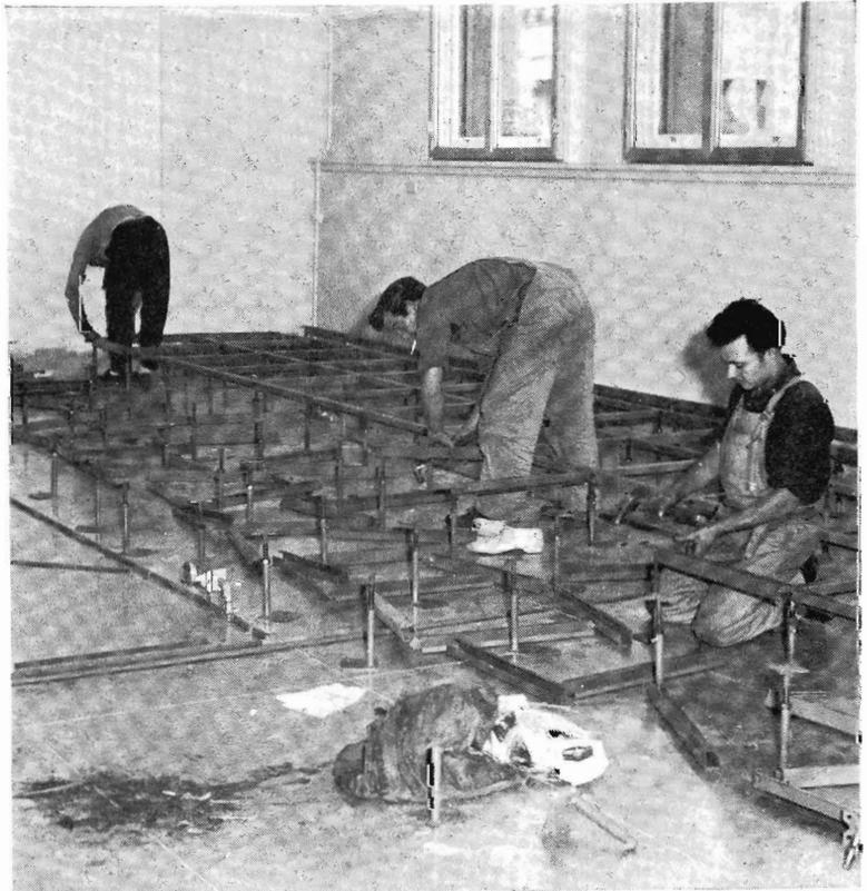
Contractor's staff are installing the sub-floor in the room that will house the computer assembly.
