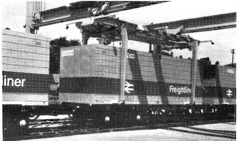
A 27-ft. container on British Railways. Note frame arranged to lift container from the bottom.
