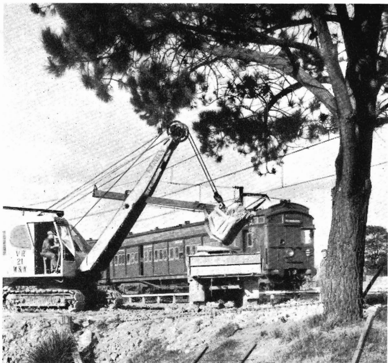
Removing earth from embankment of old Outer Circle line near Eastmalvern.
