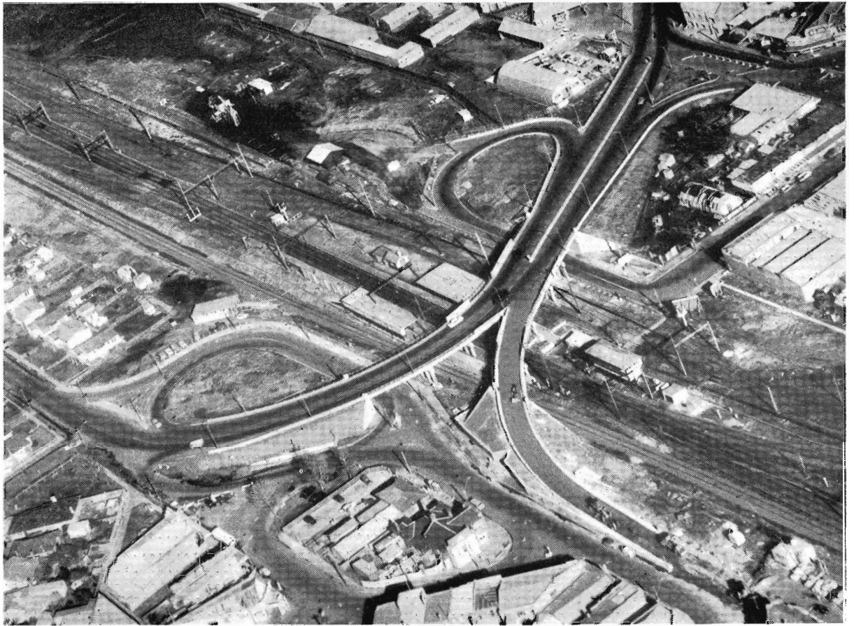
AERIAL VIEW of the Hampshire Road overpass at Sunshine. Practically a complete cloverleaf arrangement, this complex overpass crosses five broad gauge tracks, the standard gauge line and two connecting roads. (Country Roads Board photograph)
