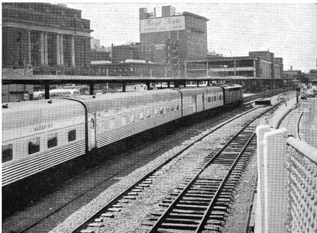
SOUTHERN AURORA glides into No. 1 platform, Spencer Street for the first time on December 13 after the platform was extended by 650 ft. to 1,150 ft. The platform, with dual guage tracks, will eventually be 1,355 ft.
