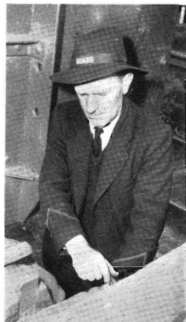
Goods Guard G. Barbour puts air through brake hose pipes of No. 5 goods
