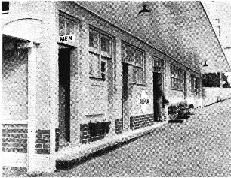
Laburnum station, between Box Hill and Blackburn, was opened in 1958. The construction of additional stations between existing suburban stations is a great convenience to local residents, but the financial return to the Department seldom justifies the capital outlay.
