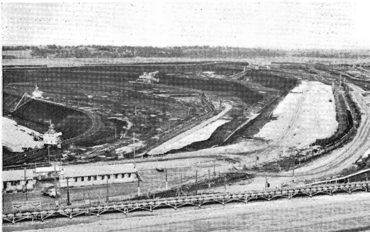
Portion of Yallourn brown coal open cut.
