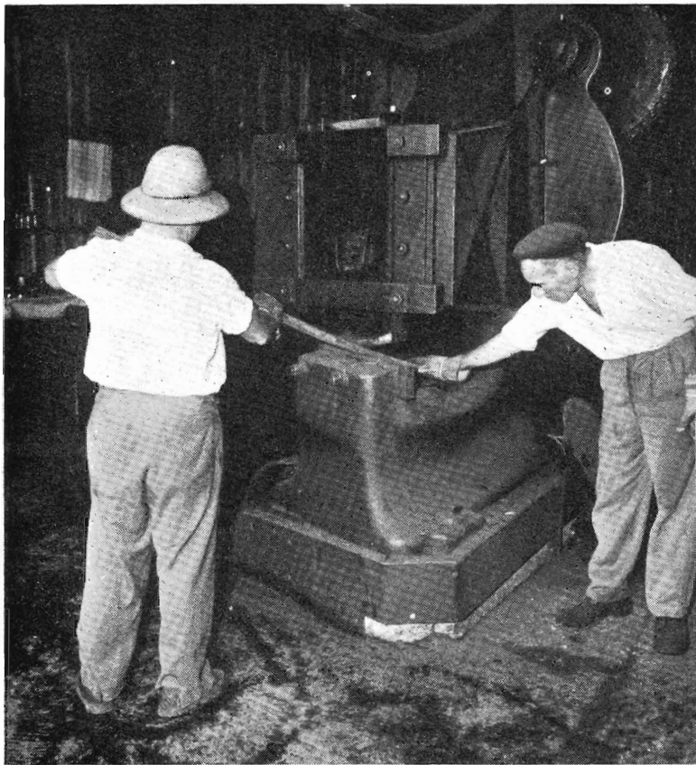
Iron Machinist A. Gilbert (left) and V. Trimboli shear steel scrap to a size suitable for smelting.
