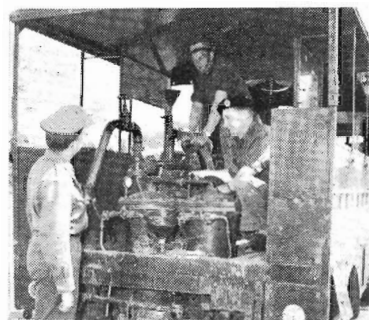
(From left): Lieutenant E. Last, Sergeant K. Withers (Sub-Foreman Ballarat Loco) and Staff Sergeant R. Binder (Safety Officer) prepare a portable water purification and pumping plant.
