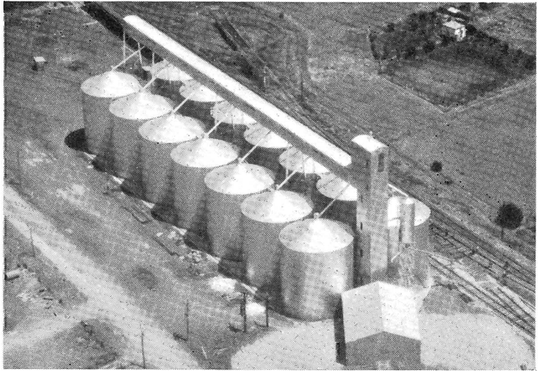
This new million-bushel steel silo at Quambatook is one of eight being built at rail sidings for the Grain Elevators Board. (Photo. Ascom Pty. Ltd.)
