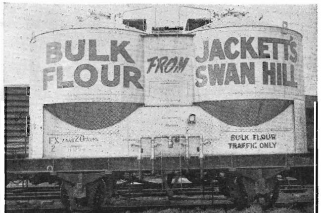
TWO JOBS IN ONE : One of seven special wagons that carry the consignor's flour in bulk and advertise it at the same time. The wagons are discharged pneumatically.
