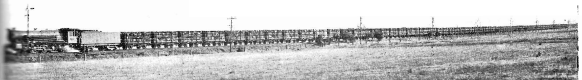
The heaviest and the longest sheep train ever run in Victoria—72 loaded trucks, containing 7,701 sheep, weighing 1139 tons and extending for more than one-third of a mile. Automatic couplers made the feat possible. Story on page 3.
