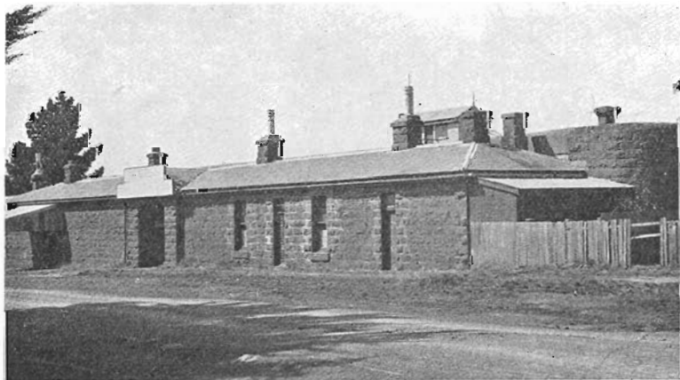
Kilmore's butter factory, just opposite the station, was once a jail
