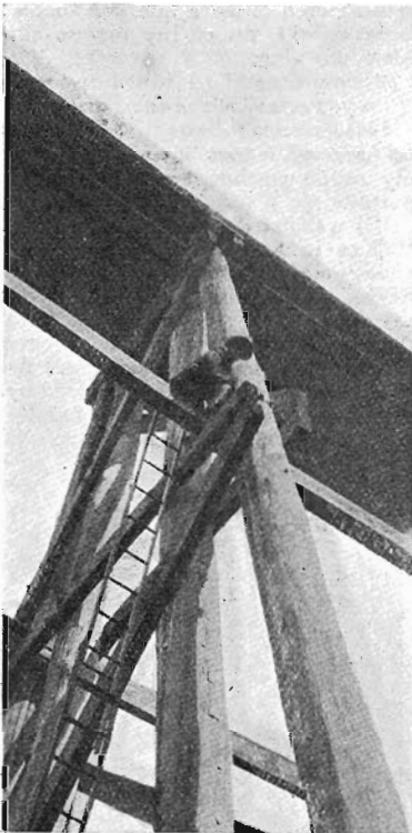
Testing a 70-foot bridge pile. Balanced on a crosspiece, the engineer is searching for possible flaws in the timber
