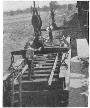
Lifting the new approach span into position.
