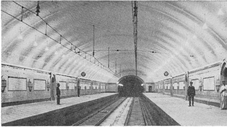
Museum station is built beneath the south-western corner of Hyde Park
