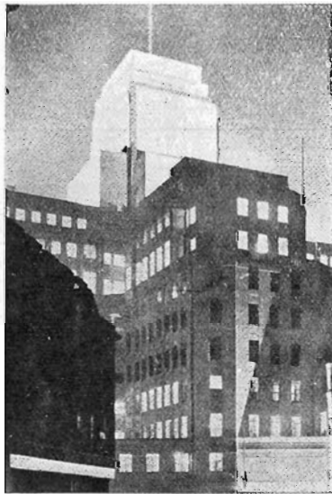
Flood-lit at night, the new St. James's Park Station which is the headquarters of the London Underground Railway, is now one of the sights of the metropolis.
