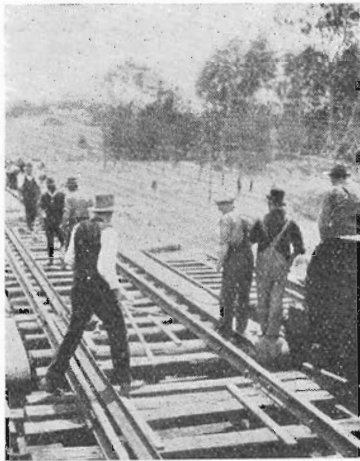
Preparing to break the track before moving the old bridge.
