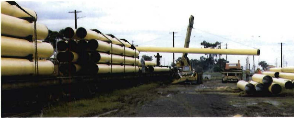
Unloading pipes at Somerton for the Melbourne-Albury natural gas pipeline.
