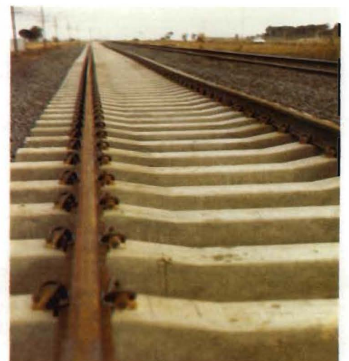
Pre-stressed concrete sleepers are being used on Sunshine-Deer Park West duplication.
