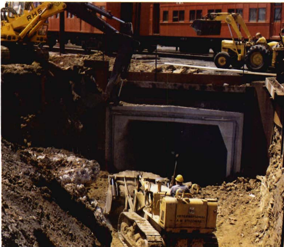
Excavations for construction of the Underground advance at Spencer Street.
