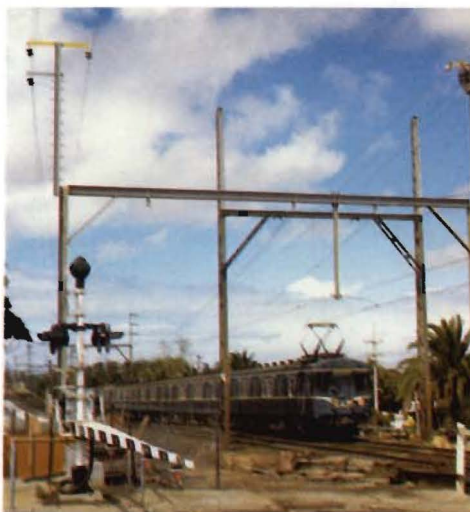
Boom barriers installed in conjunction with third track project at McKinnon.
