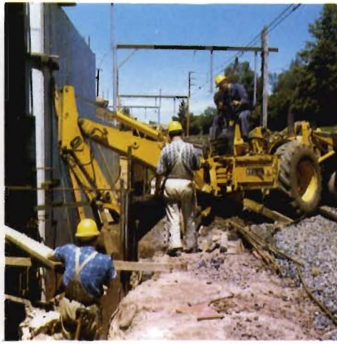
Construction works at Moorabbin for third track project.
