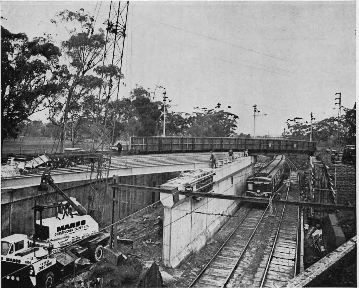
New Swan Street bridge between Burnley and Hawthorn.
