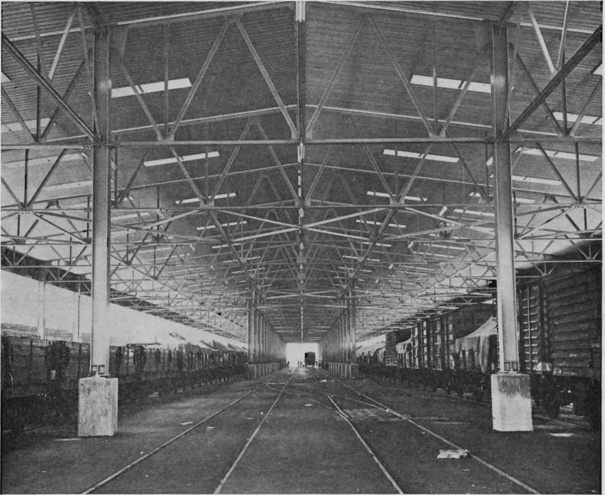
Interior view of the reconstructed No. 3 goods shed, Melbourne Goods.
