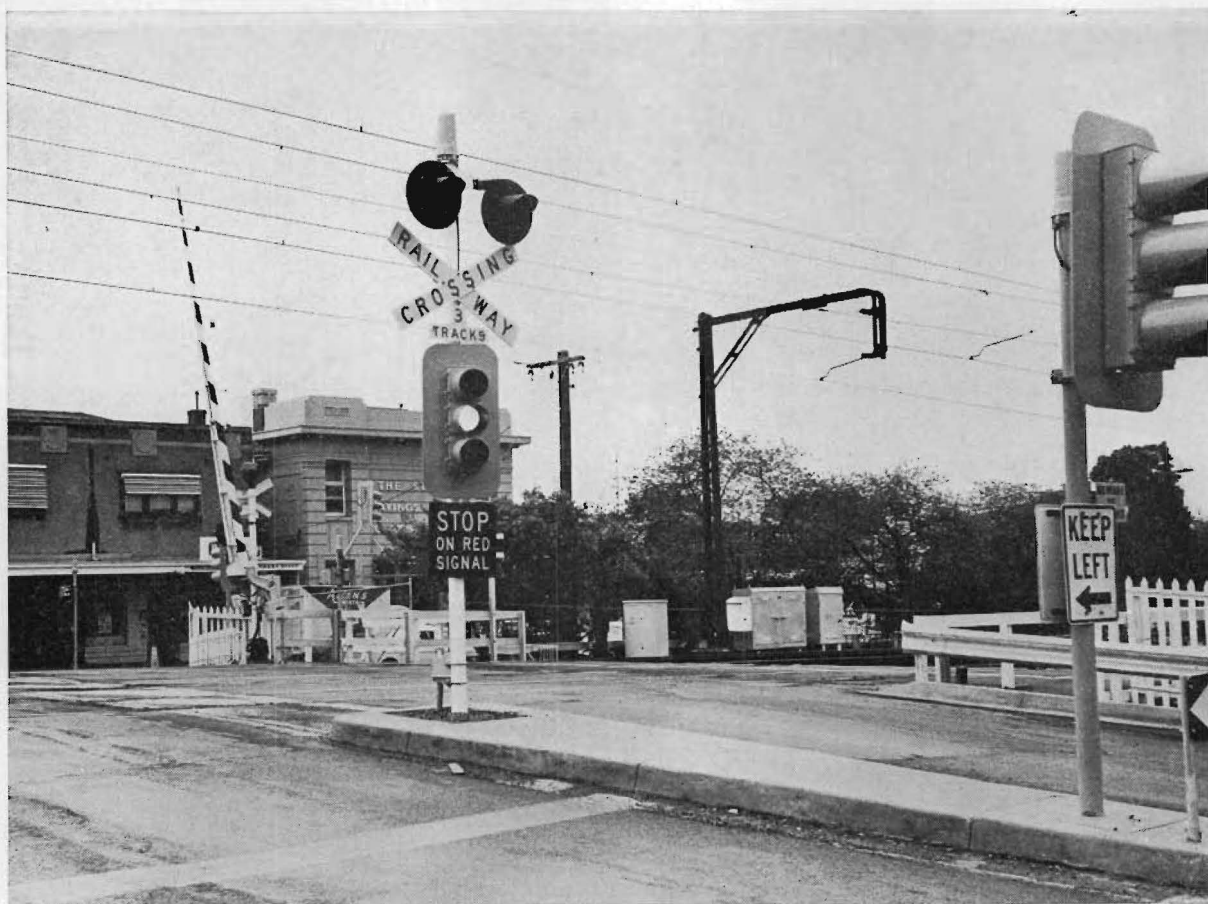
Boom barrier installation Blackburn Road, Blackburn.
