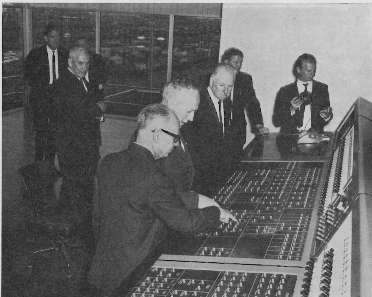
In the signal box at West Tower, Mr. Commissioner Reynolds (nearest camera) indicates to the Honorable V. F. Wilcox, M.P., Minister of Transport, some features of the push-button signalling system.
